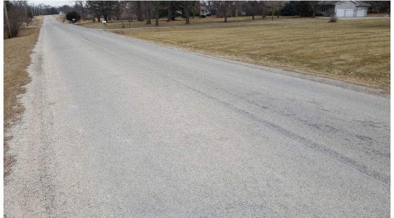
MC-3000 Seal Coat was applied over the crushed stone road approximately two years prior to the picture for dust suppression. Weather and traffic have turned the Seal Coat to a grey color with minimal dust. Proper maintenance by the owner may result in a long-lasting product.
